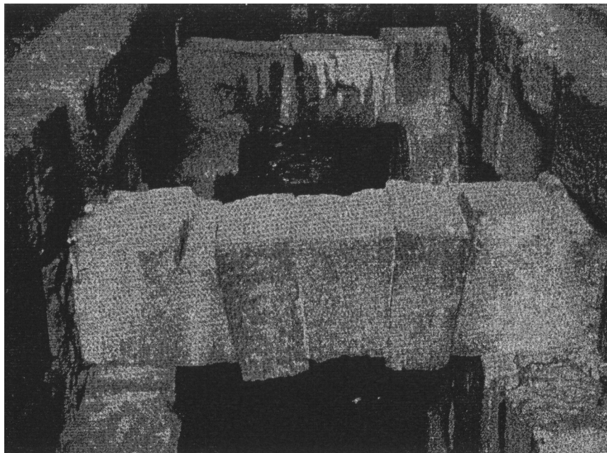
Fig. 2.12 Flat arches at the Colosseum, Rome, 1 st Century AD.
